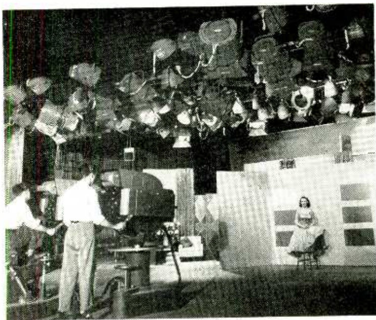
COLOUR TELEVISION STUDIO, claimed to be the first one built specifically for colour, and recently put into operation by the National Broadcasting Company of America at Burbank, California. An elaborate lighting system with 2,400 controls permits the pre-setting of lighting for ten scenes and also ten changes of lighting within any one scene. An unusual feature is an "audience pit" which accommodates the studio audience below floor level to avoid interference with the cameras.
